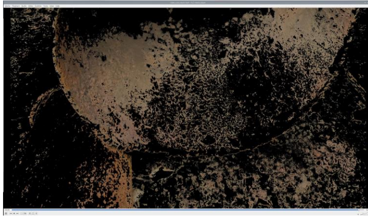
Fig. 3. A fragment of the saved video for the investigated area of corrosion on metal after applying filters in Raspberry Pi
