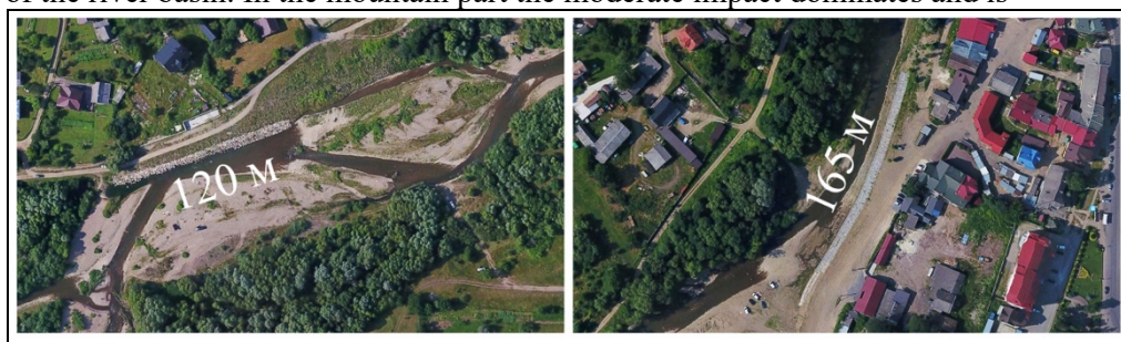
Fig. 8. Erosion-resistant constructions in Bolekhiv town
