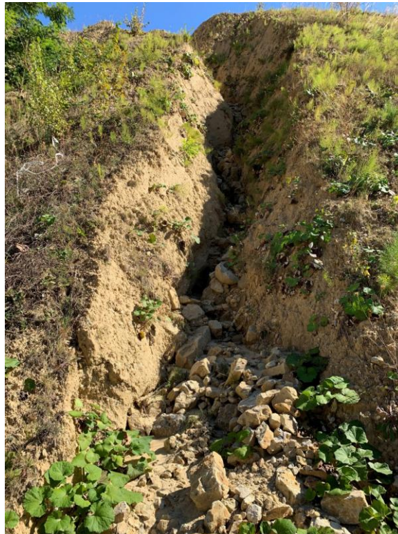
Fig. 4. The lower part of gully and the debris cone on the slope of dump (the Vynnychkivskiy Quarry)
