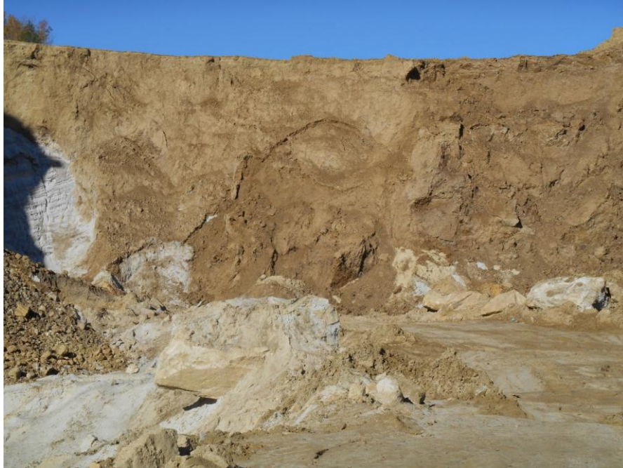
Fig. 10. Slides in heaped deposits of the Vynnychkivskiy Quarry
